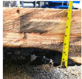
Charring tests on CLT elements. CLT char fall-off (also known as delamination) is the subject of ongoing research.
